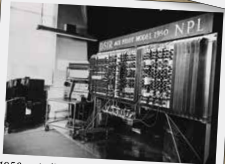
1950 – A pilot model of the Automatic Computing Engine (Pilot ACE) designed and built at NPL
